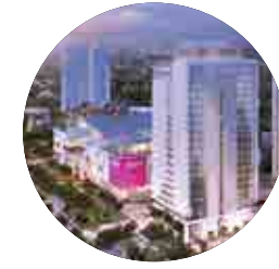
APARTMENT SOUTHGATE Jakarta
